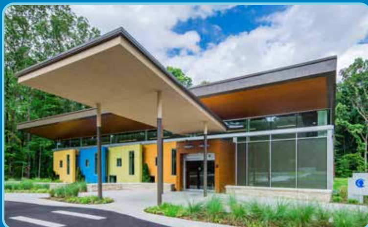
ACH SOUTHWEST LITTLE ROCK COMMUNITY CLINIC
